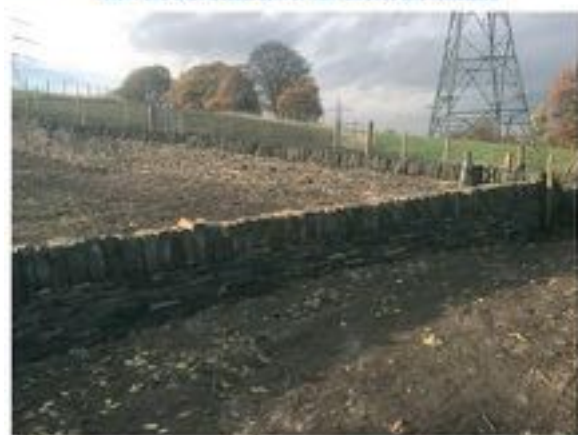
YW041 and 042 Access. 25m of wall removed and reinstated
