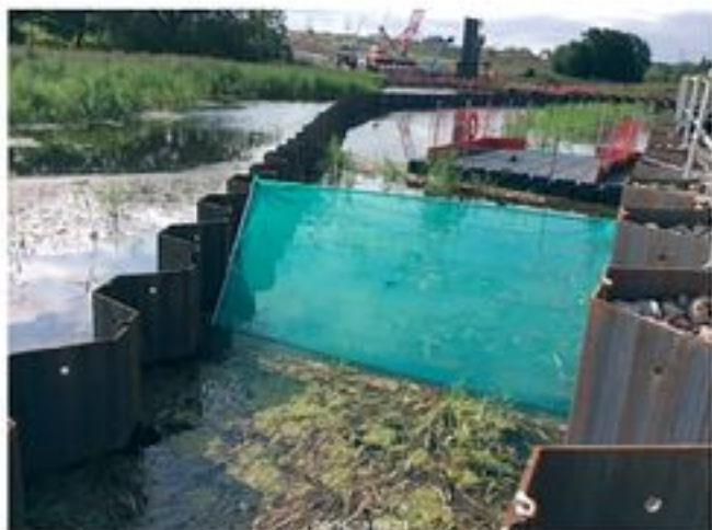
Fish Trap installed at Springhead Bridge
