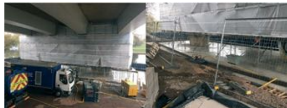
Figure 2 - Pollution prevention whilst completing hydrodemolition works Reduced plant movement and resultant air emissions through use of the Air Skid System
