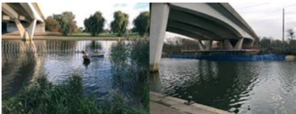
Figure 1 - Portadam installation showing minimally invasive nature of works
