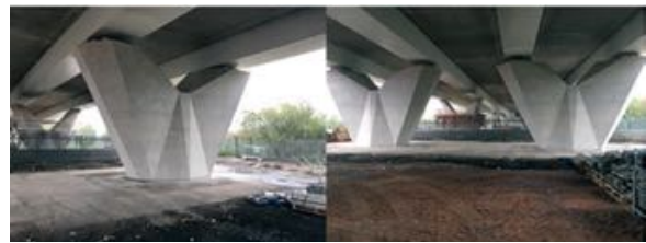
Figure 5 - Photos of completed reinforced concrete jackets
